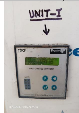
Photo 10: Inlet flow meter (unit-1&2)
