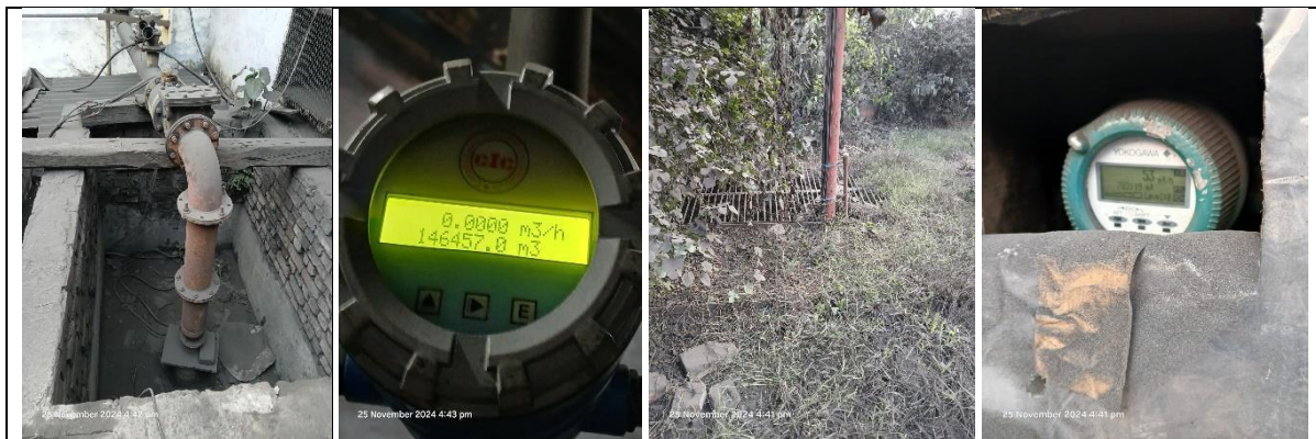
Photo 9: Borewell 1 & 2 (with flow meters)
