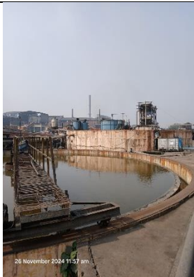
Photo 7: Secondary Clarifier (Unit-1 & 2)
