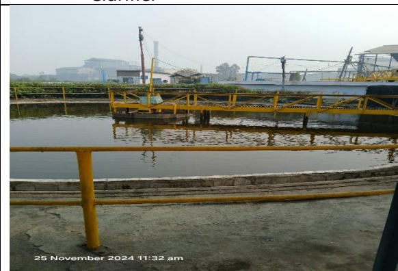
Photo 6: Secondary Clarifier
