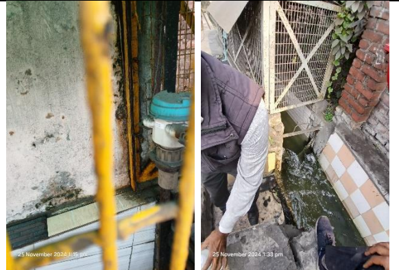
Photo 6: ETP outlet channel (Unit-1 & 2)
