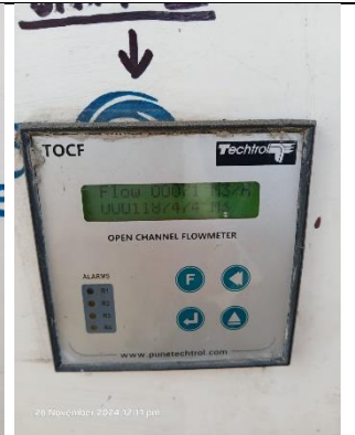
Photo 10: Inlet flow meter (unit-1&2)
