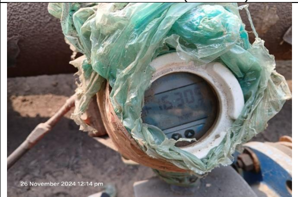
Photo 12: Flow meter at recycling line from primary clarifier (Unit-2)
