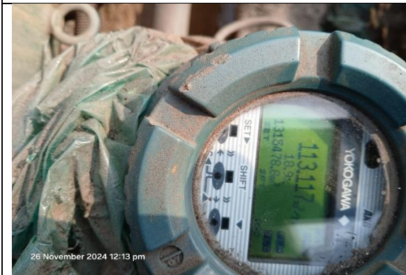
Photo 11: Flow meter at recycling line from primary clarifier (Unit-1)
