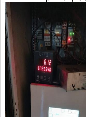
Photo 13: OCEMS and flow meter at ETP-1 outlet
