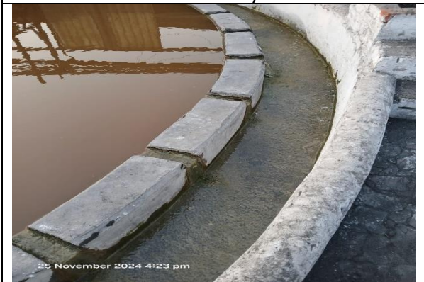
Photo 5: Secondary Clarifier
