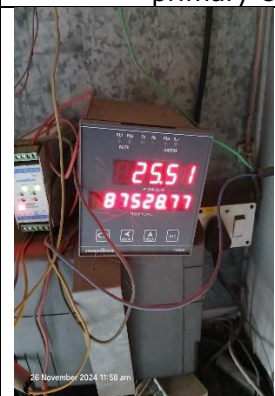
Photo 14: OCEMS and flow meter at ETP-2 outlet
