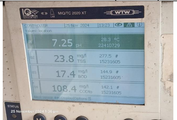
Photo 8: OCEMS at ETP outlet (unit-2)
