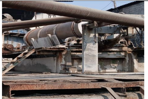
Photo 4: B2 thickener (plastic separation from effluent)
