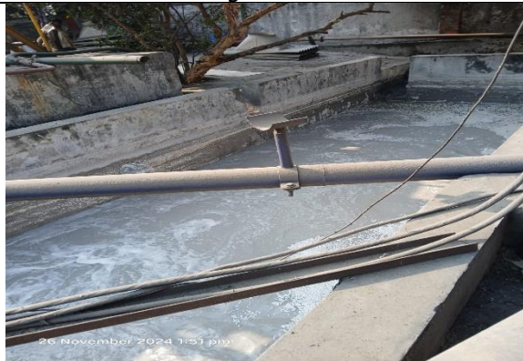
Photo 3: Equalization tank
