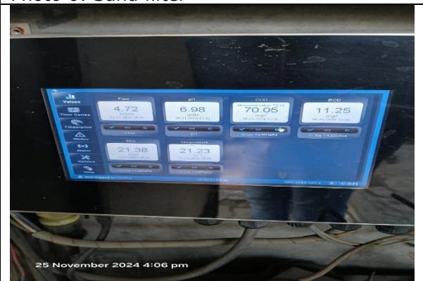
Photo 8: OCEMS at ETP outlet
